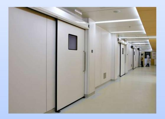
• Hermetic doors, which are used in specific application areas such as operating theaters, laboratories and even recording studios that require sealing, close with full contact on the wall and floor and meet the air tightness requirement at the desired level.
